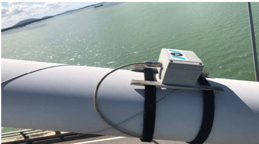
Figure 2. Accelerometer placement on cable.
